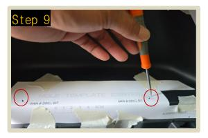
Use a center punch to mark where you'll be drilling on the center hole template.
